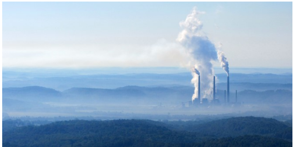
AEP's Conesville Power Station © Delta Whiskey, Creative Commons
